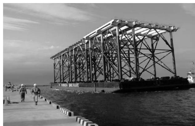
Photo 1 Jacket structure on barge
